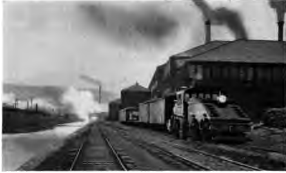
Inter-Works Line connecting various Works at East Pittsburg, Wilmerding and Trafford City
